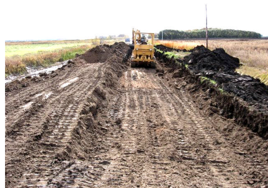
Allegra Road under construction
