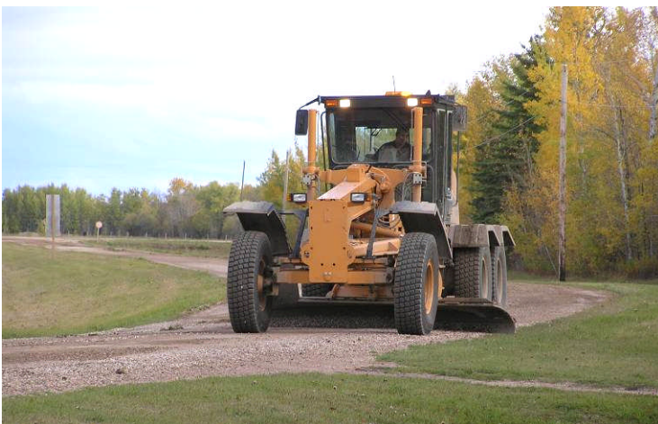
Grader Operating on a Municipal Road
